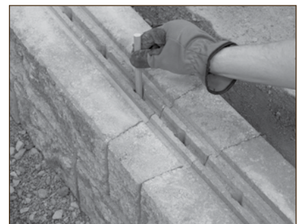
Diagram 4 - Pin Placement (Vertical Channel)
